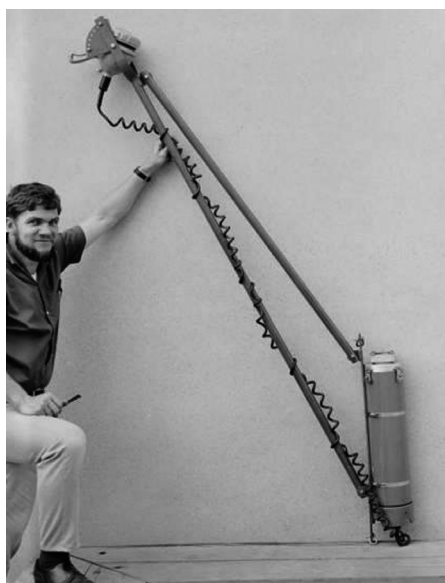
Fig. 1. The 'monster camera'. In this image the camera housing is inverted at the bottom right and the strobe is at the top left. The system was deployed with the camera facing down, towards a perforated metal can containing the bait. Photo courtesy of Scripps Institution of Oceanography Library
